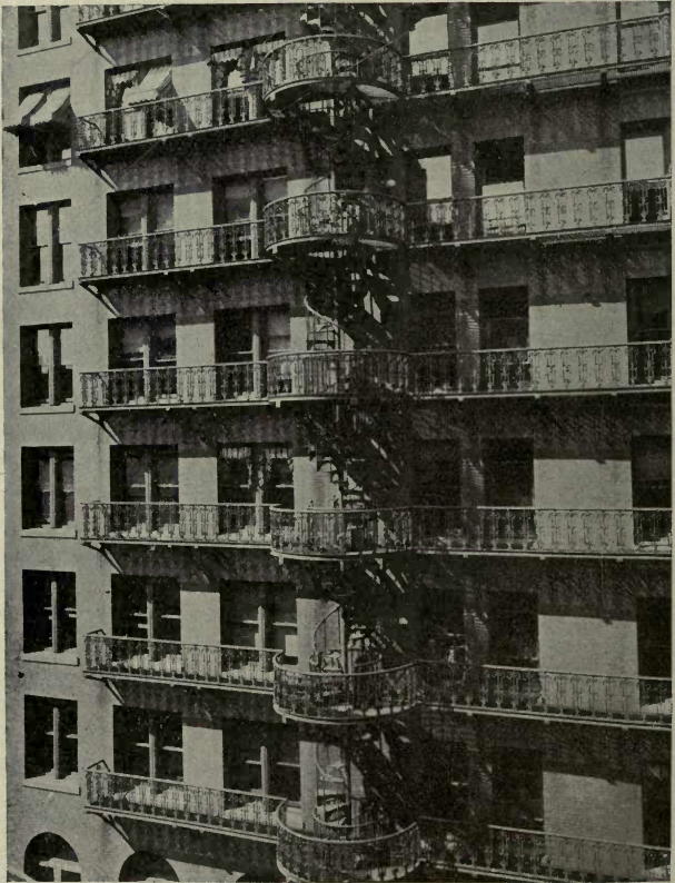
FIG. 183. — Circular Stair Fire Escape, Pemberton Building, Boston.
